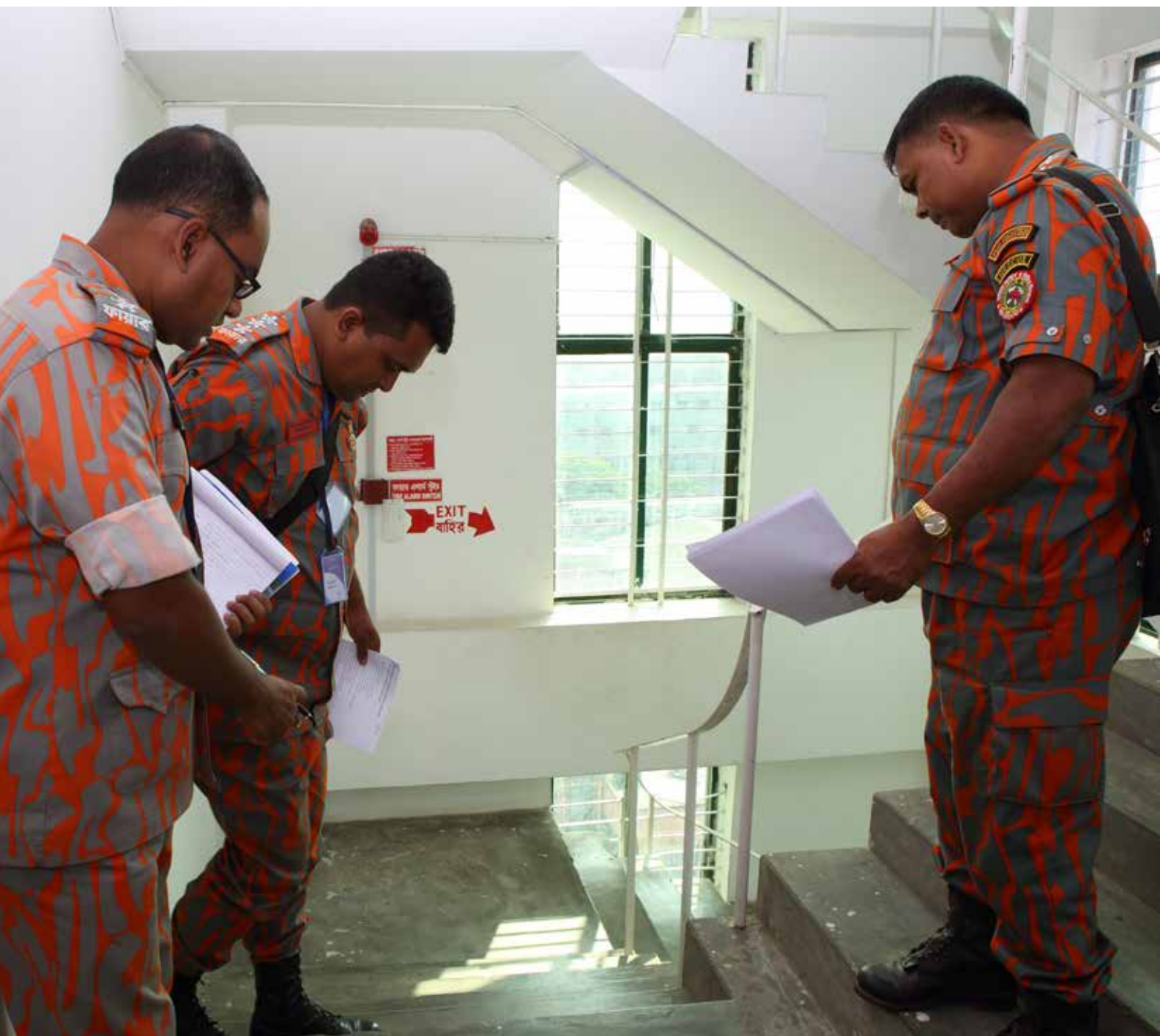
Fire inspectors check an exit stairway in an RMG factory.
